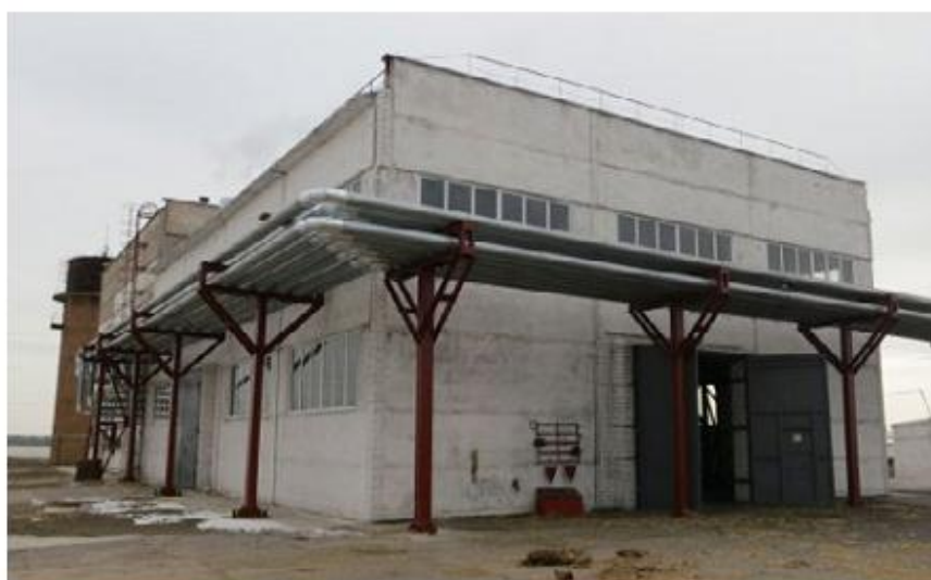
Fig. 4.4. 10 MW boiler plant running on baled straw at Dniprovsky battery farm (Pershotravneve village, Nikopolsky district, Dnipropetrovsk region) 55 .
