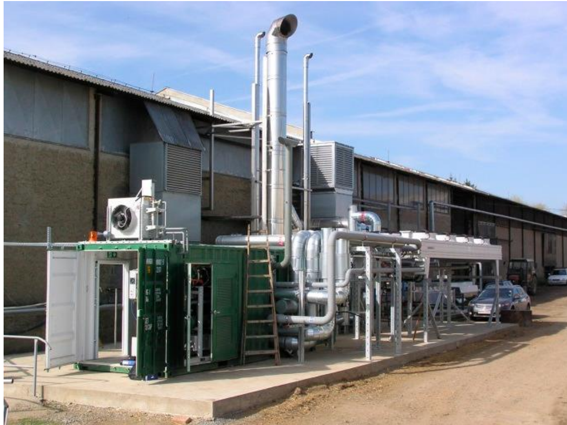
ORC system (using R245fa) of a biogas plant in Dublovice, Czech Republic
