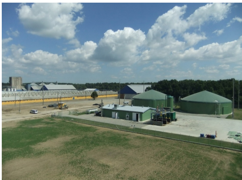
Fig. 3.5. Biogas plant at «Danosha Ltd», village Kopanky, Ivano-Frankivsk region
