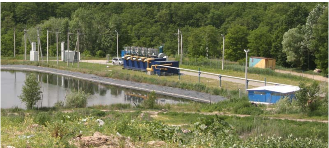
Fig. 3.7. TEDOM biogas engines with capacity of 5×177 kW e at the landfill #5, Kiev region
