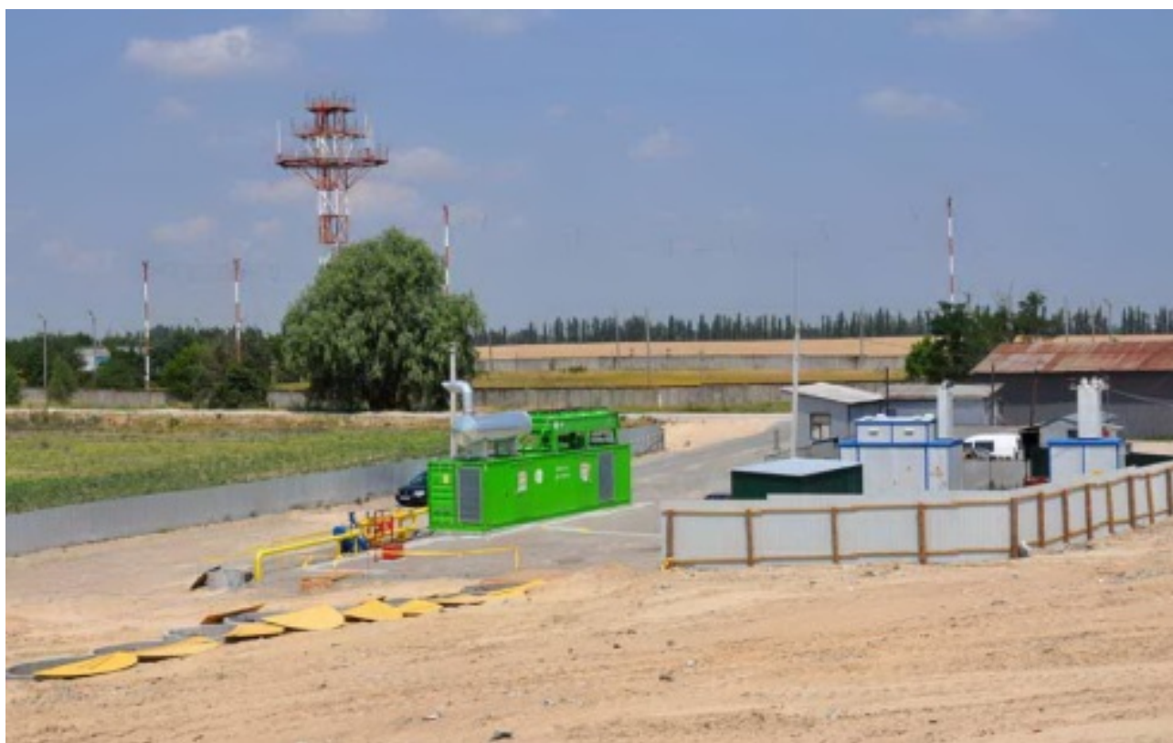
Fig. 3.8. Biogas engine GE Jenbacher with capacity of 1063 kW e at Boryspil landfill
