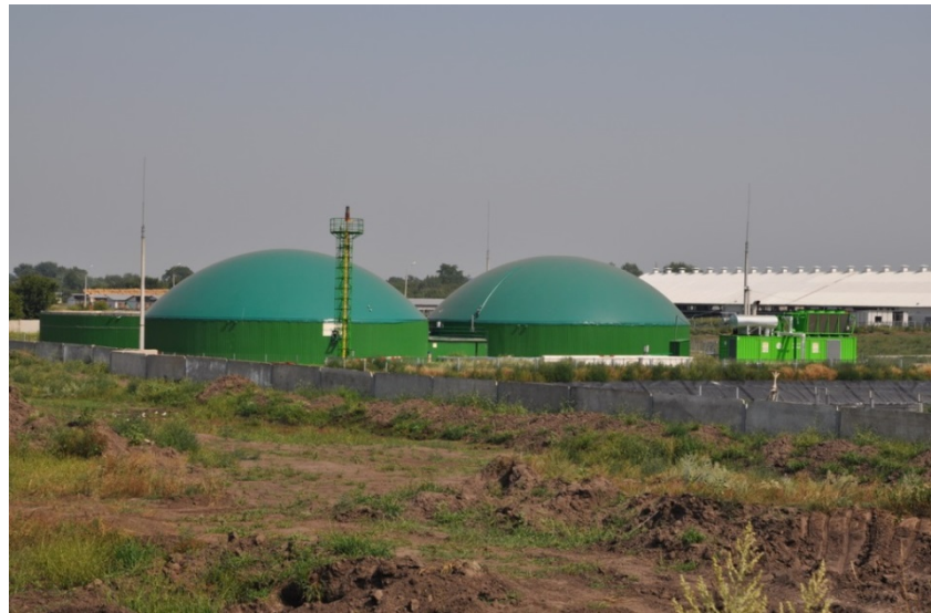
Fig. 3.3. Biogas plant at cattle farm of "Ukrainian dairy company", Velykyi Krupil village, Kiev region
