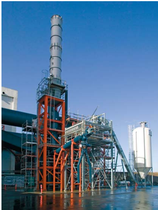
The gasification plant in Kalundborg, where the straw is converted into gas before it is burnt at the nearby power plant.
