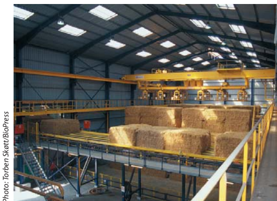
Straw storage room at the Ensted Power Station in Aabenraa. Note that the crane is capable of lifting 12 bales at a time.
