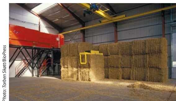
Straw stockroom at Terndrup district heating plant. The transport from the stockroom to the boiler takes place with an automatic controlled crane. The stockroom can contain straw for about one week's operation during winter.
